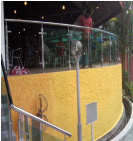
Photo 7 Poolside round wall painting and tempered glass completed.
