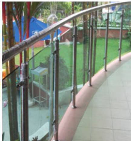
Photo 8 Completion of tempered glass at poolside bar area view
