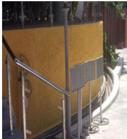
Photo 5 Completion and painting at round wall area view
