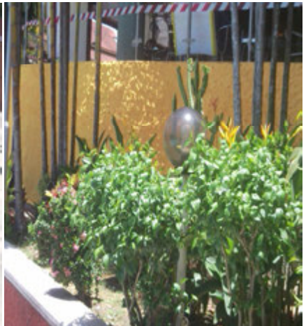
Photo 6 Completion of painting work at round cement wall area.
